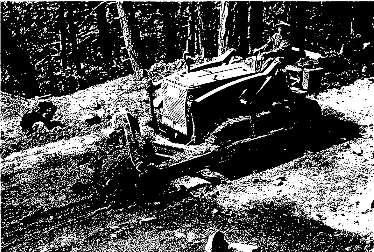
Figure 28. George Morey at work on the Mt. Reuben Road in 1933 or 1934; from George Morey Collection, courtesy Medford District BLM.
