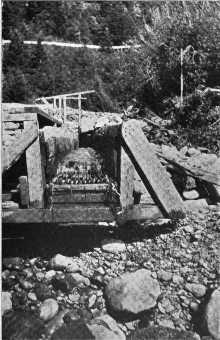
Fig. 39. Grizzly and flume of the Red River Gold Mining Company. Only the material passing through the grizzly goes through the sluice boxes
