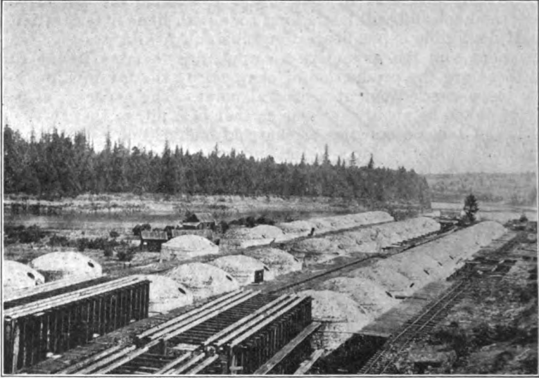
Beehive charcoal ovens at former plant of Oregon Iron and Steel Company, Oswego, Oregon
