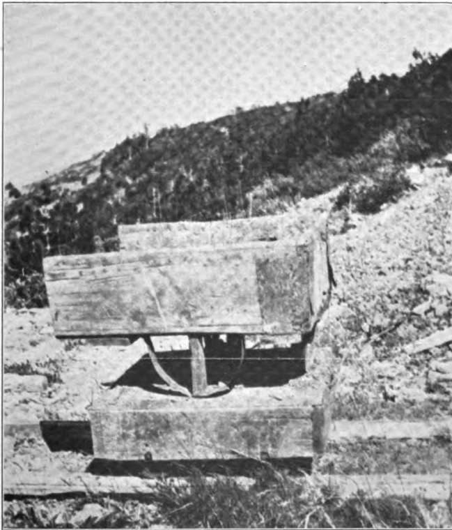
Fig. 29. Primitive dump car running on wooden rails used in driving a tunnel of the Starr (McKinley) group
