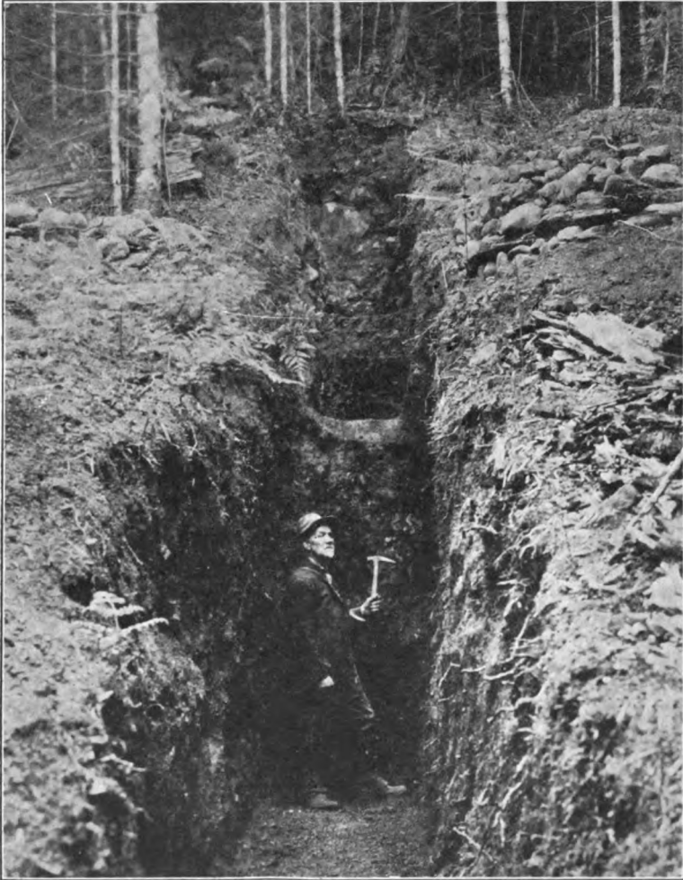
Open cut at Ironcrest. Fifteen feet of ore overlain by weathered basalt
