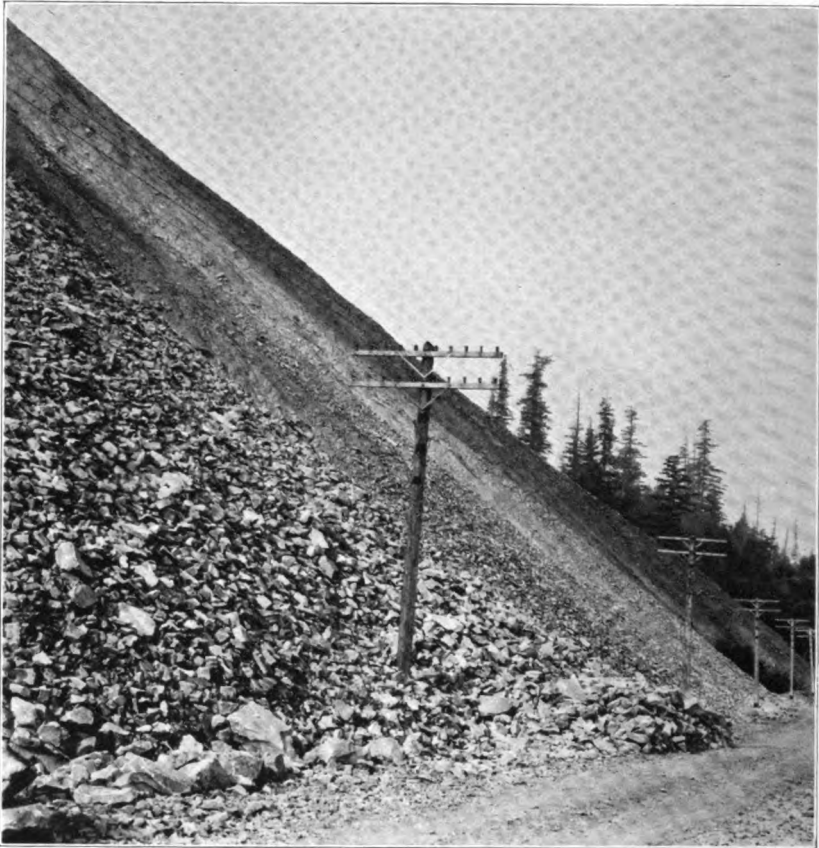
Rockslide at base of Shellrock mountain. Wherever the rock scales away, long unstable talus slopes result. In the view it is evident that constant vigilance must be practiced to maintain the road in passable condition. A hundred feet or so up we see occasional signs of the old state road whose position could not but be a notoriously insecure one
