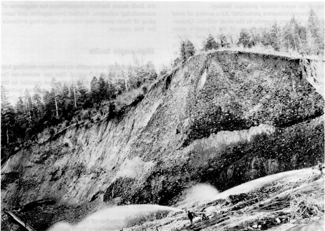
Figure 3. Old channel gravels at the High Gravel (Osgood Mine), No. 416, near Waldo. Millions of cubic yards were mined here by hydraulic methods, mainly in the late 1800's.
