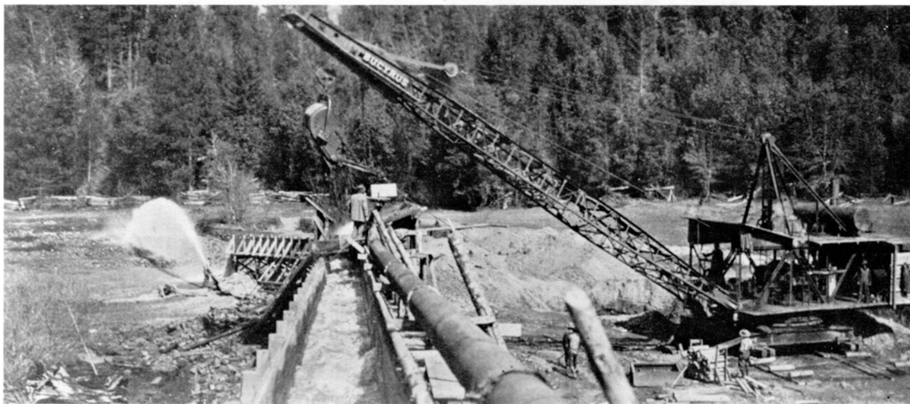
Figure 8. Sluiceway and wood-fired, steam-powered dragline at Leonard Placer Mine on lower Althouse Creek during the 1930's.
