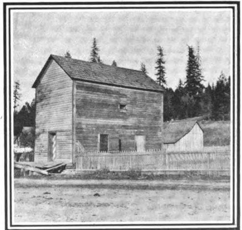
THE OLD JAIL IN KERBYVILLE—A relic of the old rough-and-ready days.
